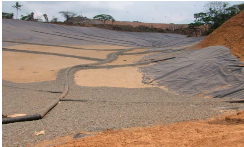
Landfill at Mangalore (Karnataka) during construction
